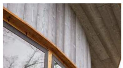
As Thermory only ships usable boards and cuts down on material waste with a number of innovative processes and solutions, there was enough material left over from the original order to sand down and repurpose the cladding boards as a natural trim. Over time, this trim and the Drift cladding will both undergo a unique aging journey until they arrive at a gorgeous, rustic silver finish.
